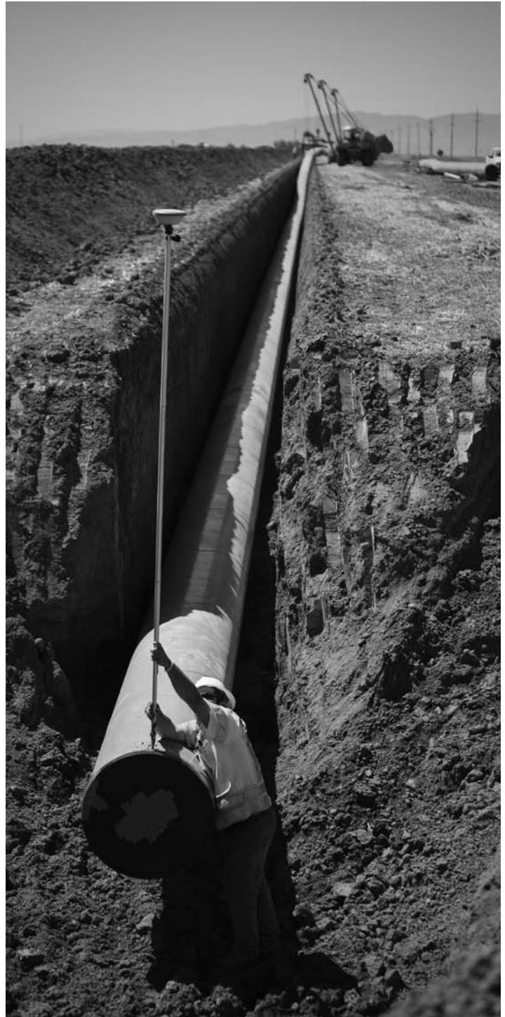
Installing irrigation pipe in California's Central Valley. Photo courtesy of Provost & Pritchard Engineering Group.
