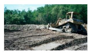
Nearly 30 miles of ditches and canals have been filled and compacted. Additionally, approximately 4 miles of earthen dike around two retention ponds are currently being leveled. Thousands of exotic Brazilian Pepper tees have been pulled and burned.
